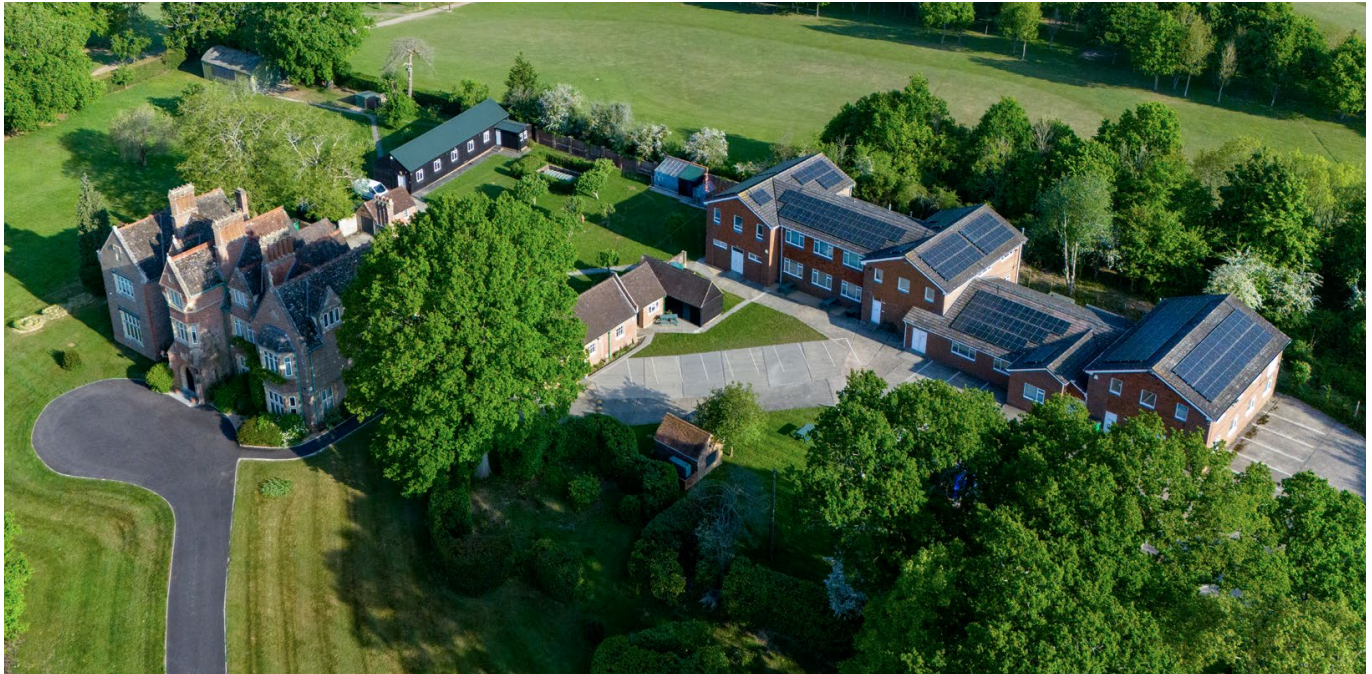
Lodge Group Headquarters
