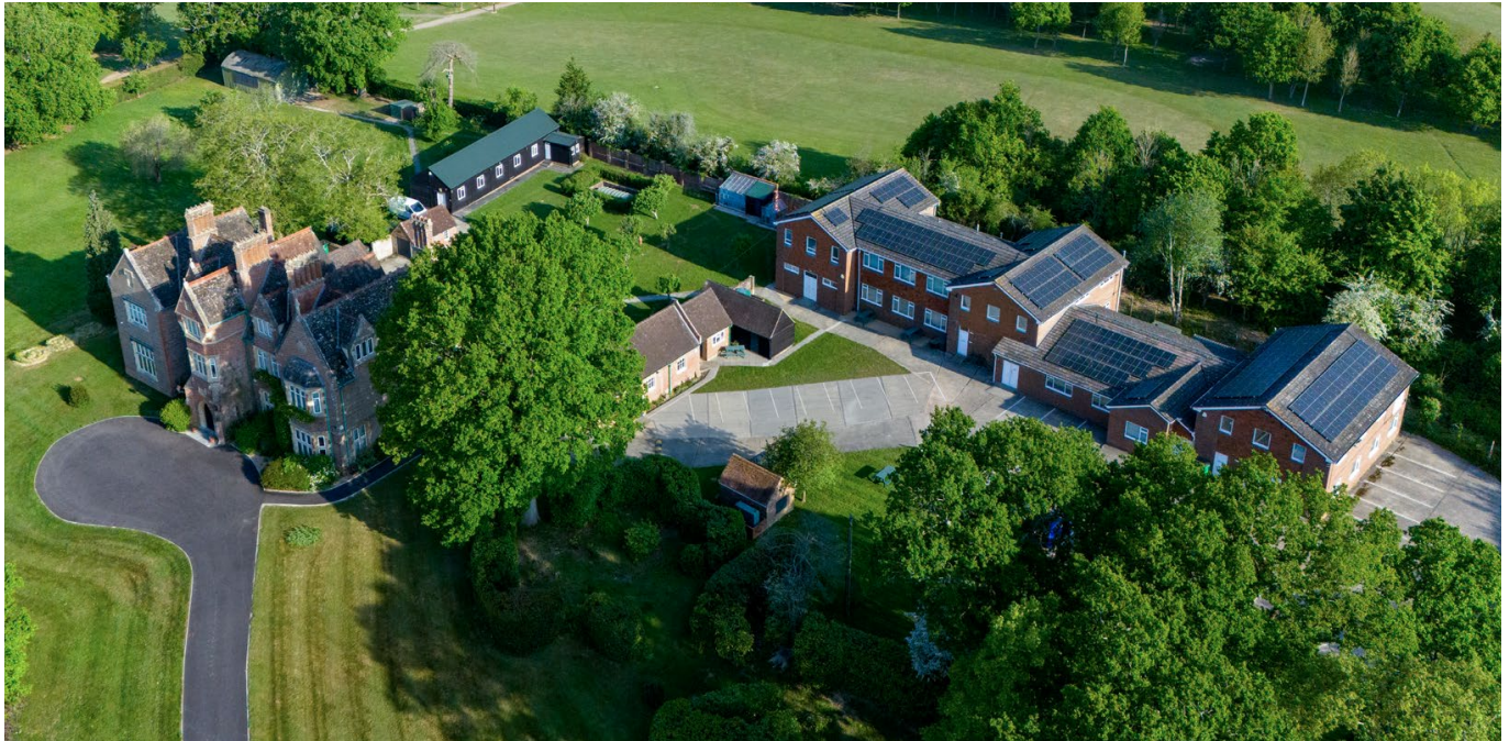
Lodge Group Headquarters
